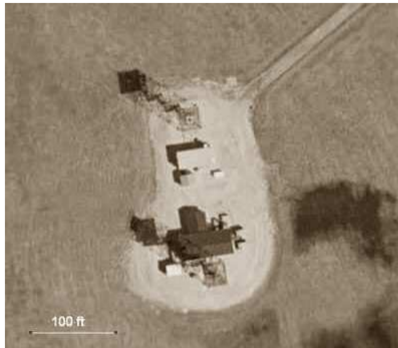
Fig. 15 Aerial View of ASR-9, ORD #1, Chicago O'Hare, Dupage County, Ill.
