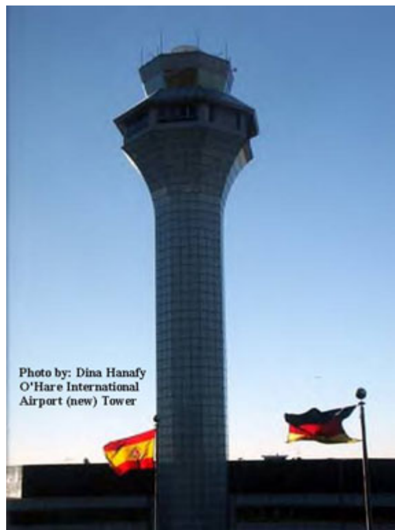
Figure 7. New O'Hare Airport Control Tower
